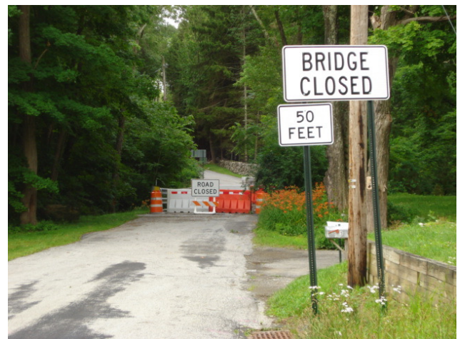
Bridge Closure Barricade & Sign Setup
