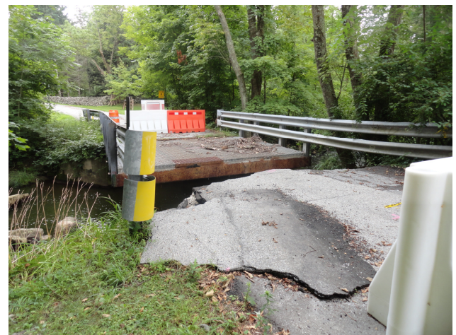
Bridge Abutment Failure
