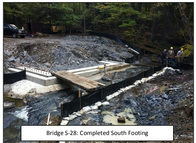
Bridge S-28: South Footing Concrete Pour
