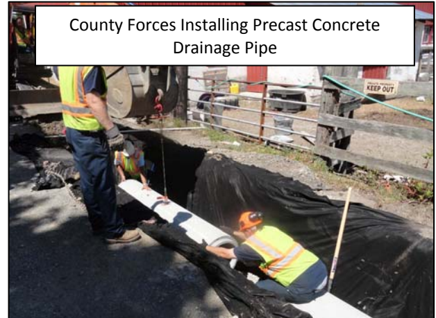
Reinforced Concrete Pipe Installed to Replace Failed Corrugated Metal Pipe Culvert and Formwork for Concrete Headwall in Progress
