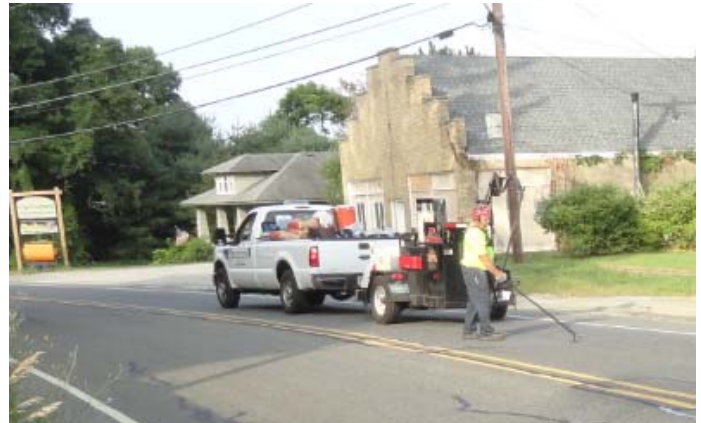
Crack Sealing CR 517 Sparta Munsons Corner Rd
