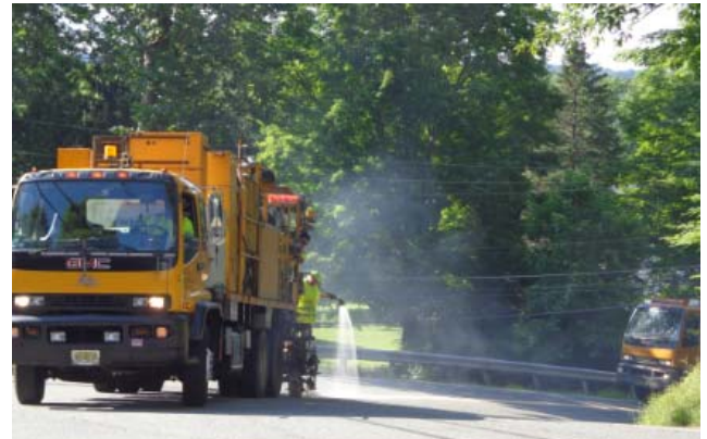
Striping Double Yellow Lines on CR 617
