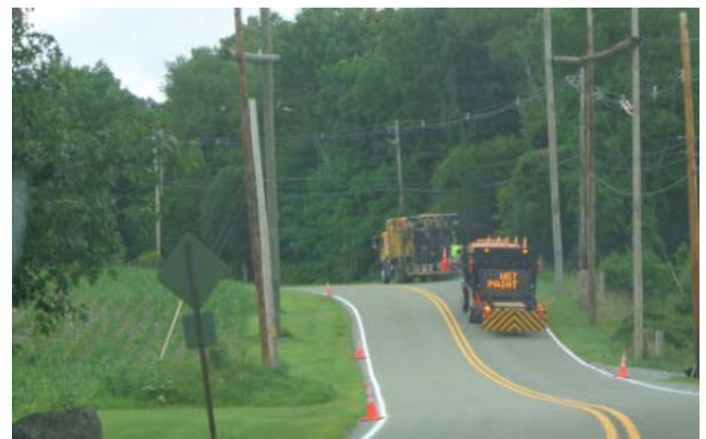
Striping White Lines on CR 617
