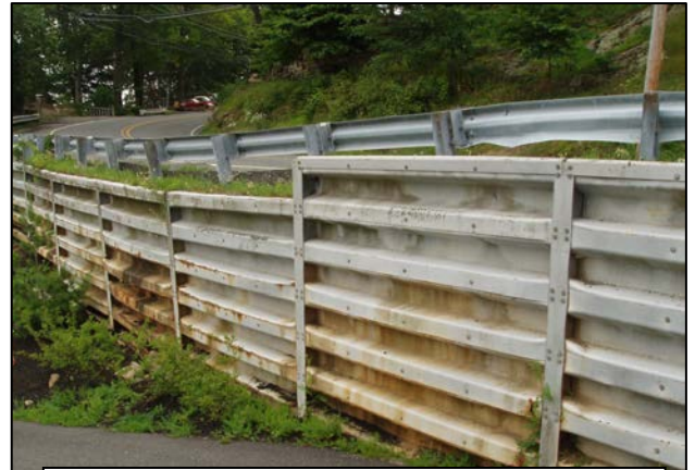
Picture of Existing Retaining Wall, CR 607 above.
