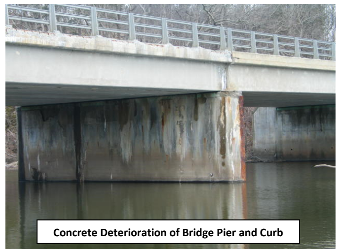
CR 642 (Owens Station Road) over Wallkill River
