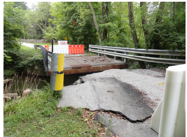
Bridge Abutment Failure
