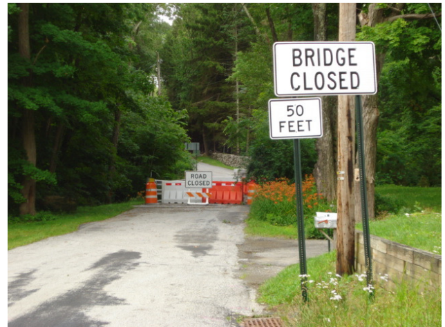
Bridge Closure Barricade & Sign Setup
