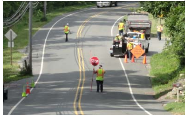
Typical Cracksealing Operation
