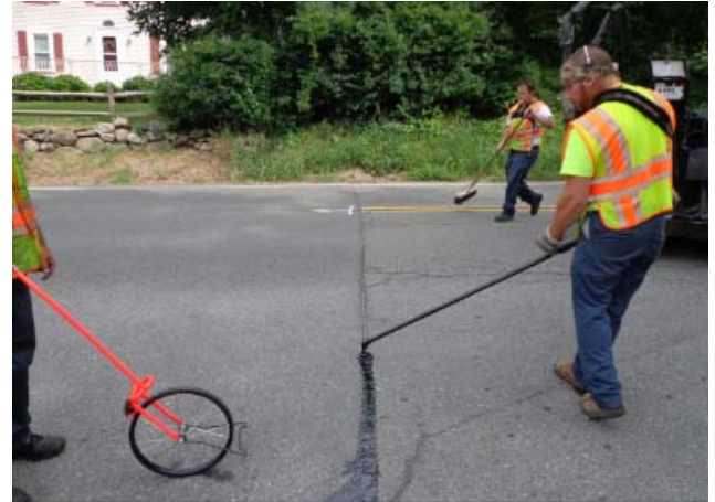
Typical Cracksealing Operation
