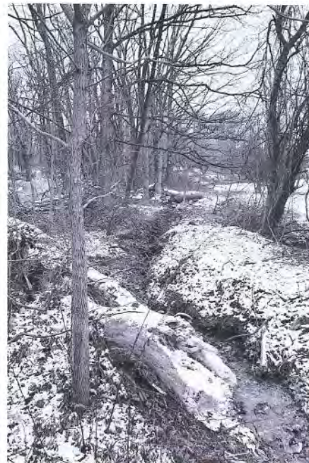
Upstream - Recently dug out by property owner - Root exposure
