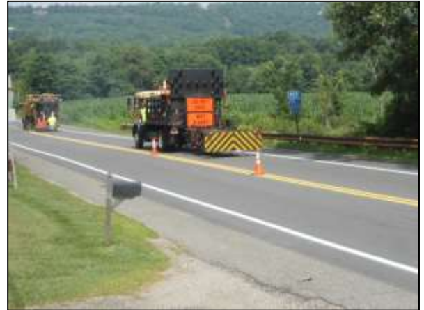
Typical Striping Operation
