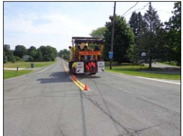
Typical Striping Operation
