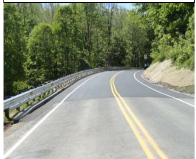
Eastbound View CR 644 Re-opened to Traffic
