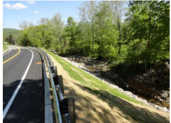
Completed Slope Remediation
